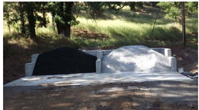
Finished road material bins September, 2011
